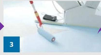
3 Coating the floor completely
